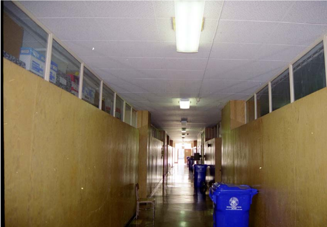
Figure 6: Classroom Building – Interior Corridor
