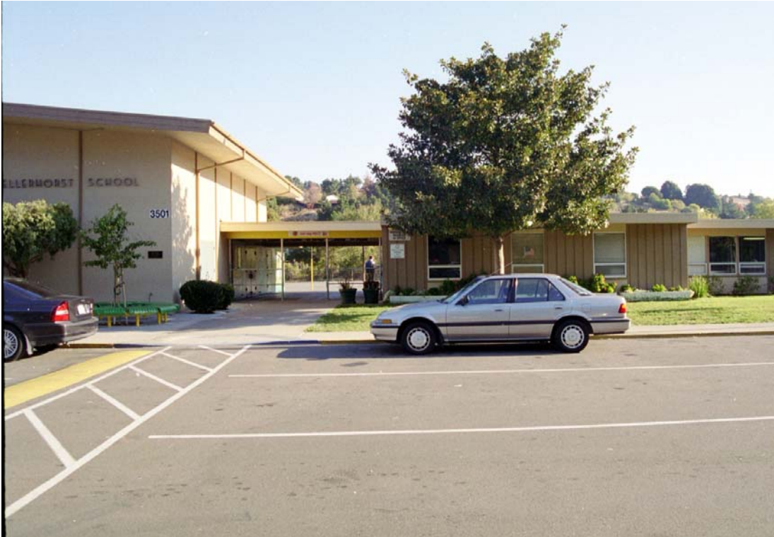
Figure 3: Multi-purpose and Administrative Buildings
