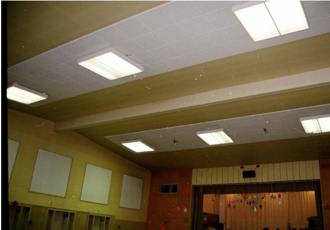
Figure 8: GluLam Beam with Crack
